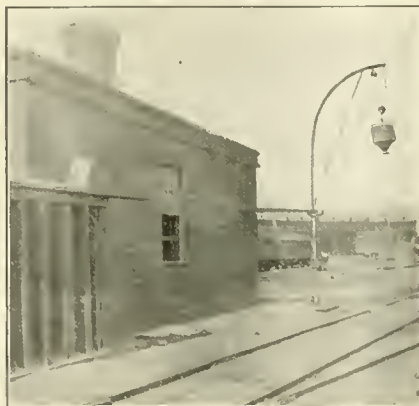
LOCOMOTIVE SAND HOIST.
